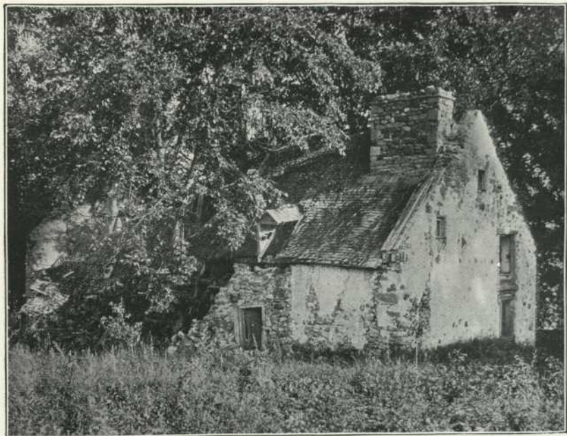
LA SALLE HOUSE OLD HUDSON BAY TRADING POST
