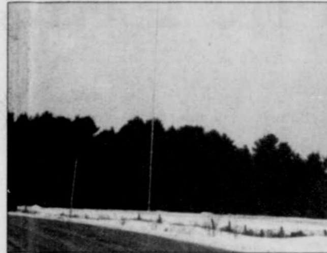
One of the windmill projects that MRC Pontiac is going to manage in the future.
