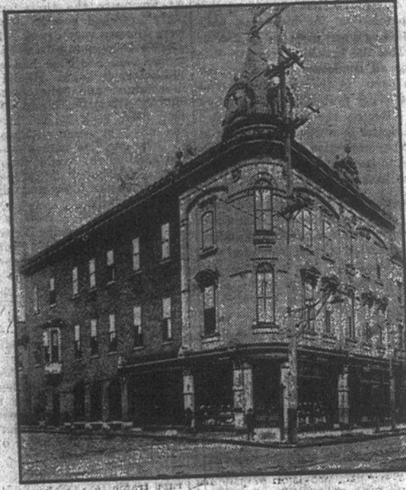
CITY AND DISTRICT SAVINGS BANK.
