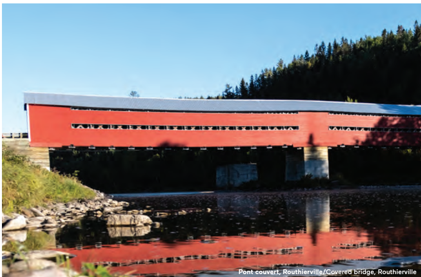
Pont couvert, Routhierville/Covered bridge, Routhierville
