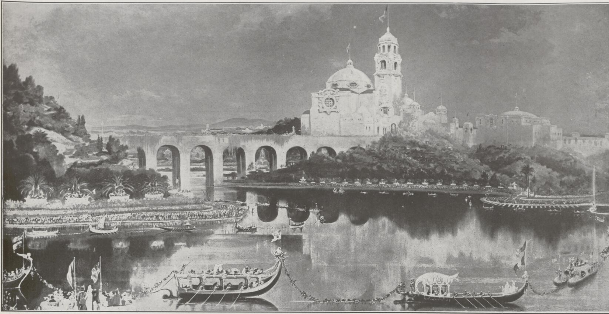
THE ALL-YEAR PANAMA CALIFORNIA EXPOSITION AT SAN DIEGO IN 1915.—The above picture shows the accepted design for the inaugural fete on the night of Dec. 31, 1914. The viaduct is 900 feet long and 136 feet high, and consists of seven arches of reinforced concrete. The lights will be turned on at midnight on Dec. 31, and at the same time a 100 gun salute will be fired by three shore batteries of four field guns and by batteries on board the flagships in the harbor. The buildings seen in the above illustration include the California State Building and the Ethnology and Fine Arts Buildings.
