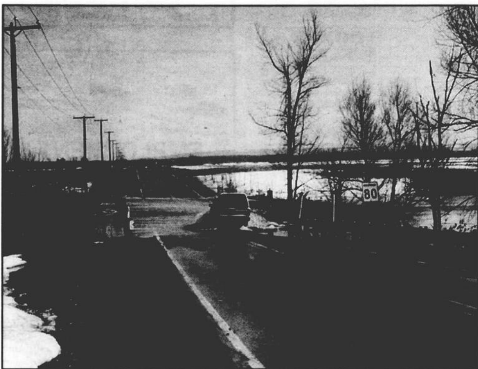
A section of Route 202 between Huntingdon and Herdman flooded last week, as it usually does, but brave motorists continued to make the crossing. (Photo: PL)
