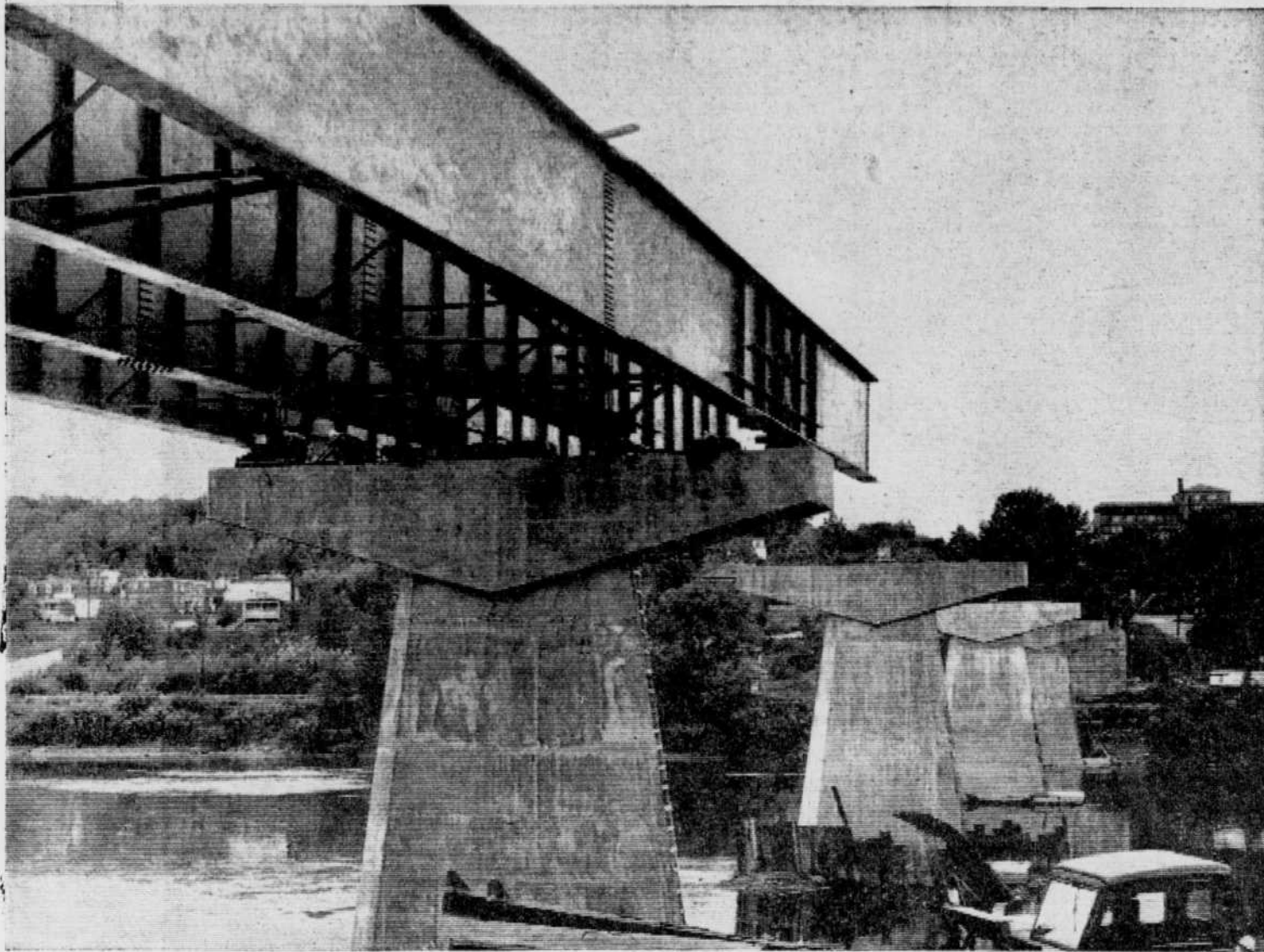
St. Francis bridge under construction
