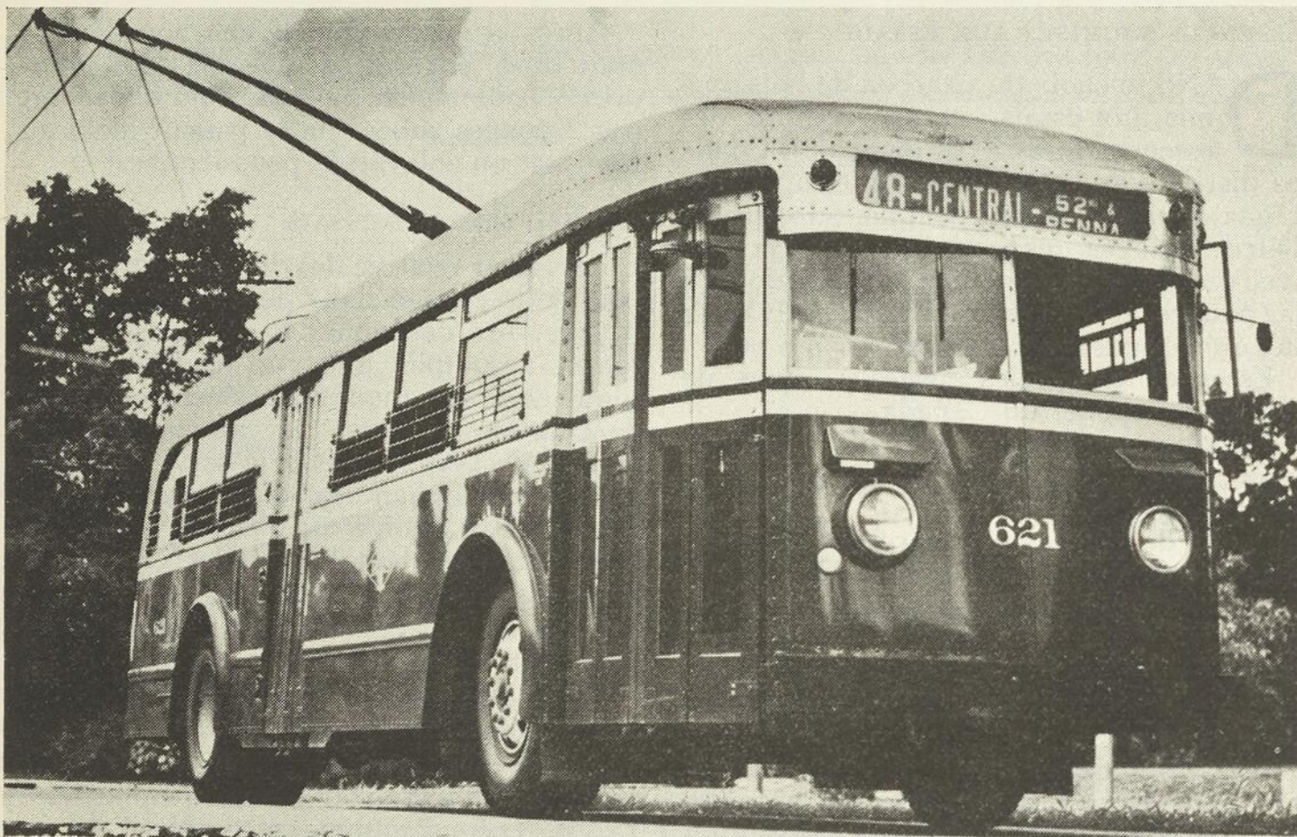
Trolley coach equipped with G-E 2-motor electric drive. In use by Indianapolis Steel Railways, Indianapolis, Ind.
