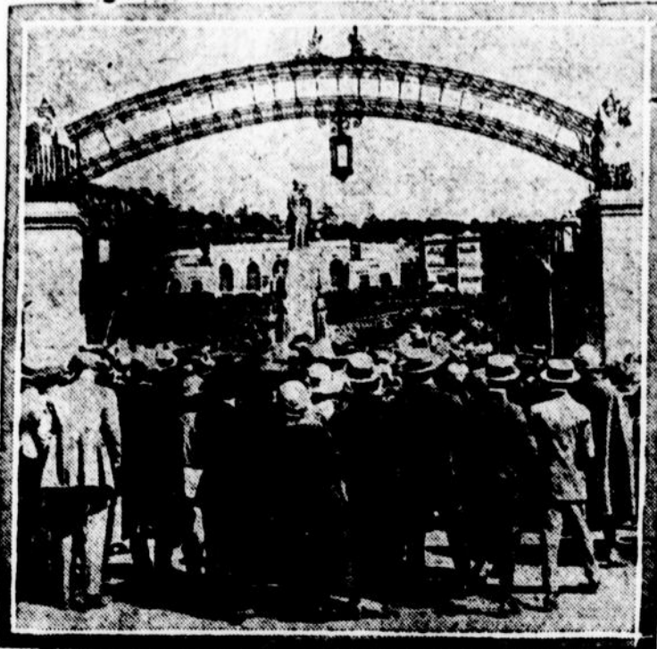
The unveiling of the statue of St. Joseph at the entrance to the famous shrine at the oratory on the slopes of Mount Royal, was attended by over twenty-five thousand people many of whom came from distant points to pay tribute to the spot built and developed by Montreal's 'Miracle Man'—Frere Andre.
