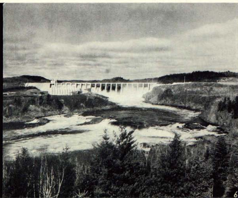
Hydro-electric plant at Chute à Caron.
