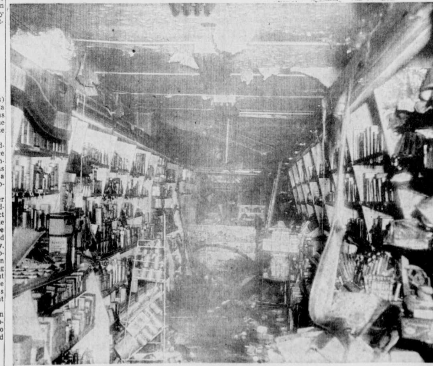
SHAMBLES IN WAKE OF FIRE — Pictured above is an interior view of the ruined Wellington Pharmacy at 98 Wellington Street, North, wrecked by flames early this morning in a two-alarm fire. Four other businesses in the same building suffered slight smoke and water damage. The fire is believed to have started in the basement below the pharmacy and spread quickly to the walls and ceiling above. No estimate of the damage was available. (Record Photo by Gerry Lemay)
