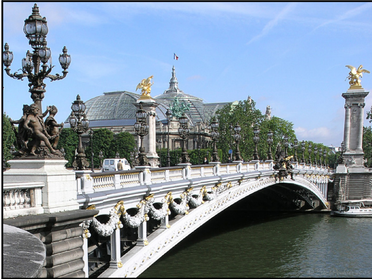
Figure 2.73: Bridge Alexander III.
