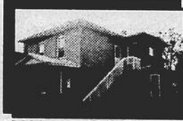
HUNTINGDON: Well located in the village duplex
