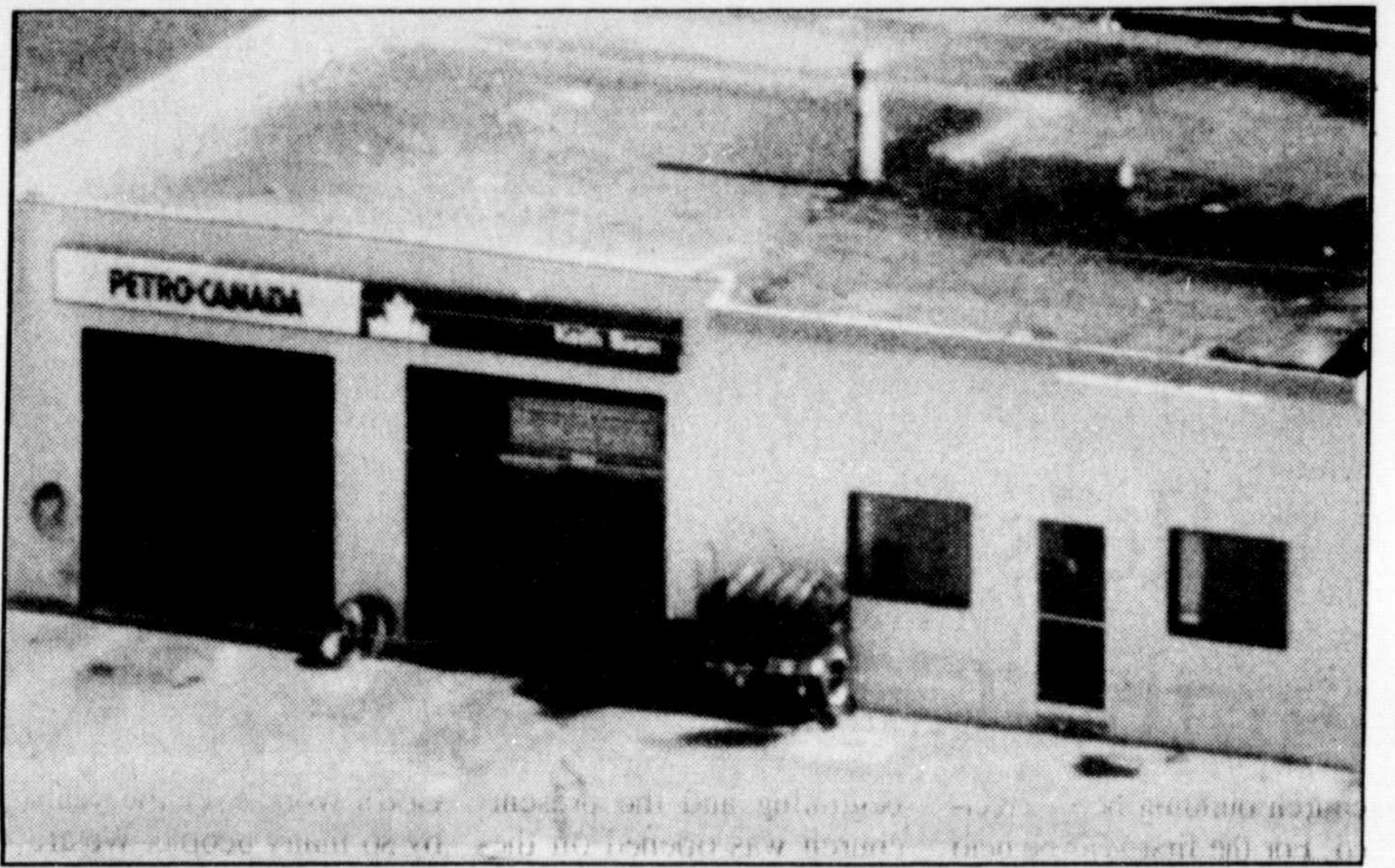
The original building only encompassed the middle section as it is known today.
