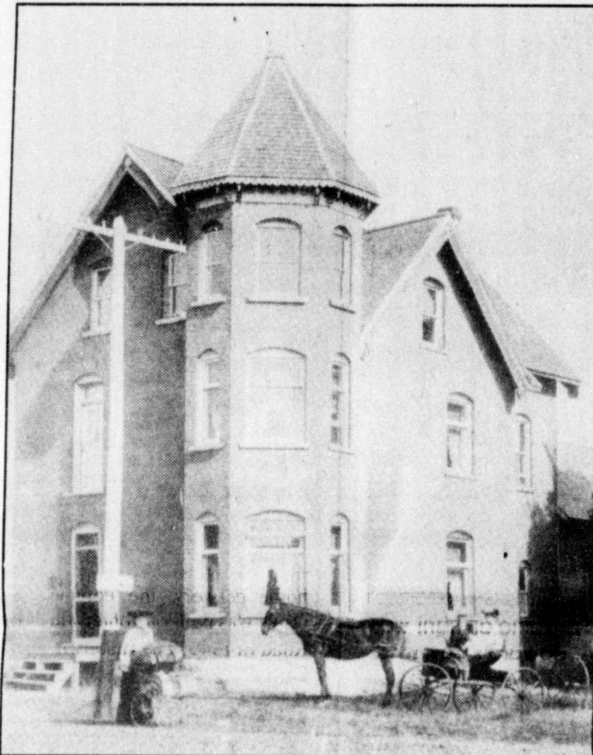
Pictured at right: The home at the corner of Victoria and Lang Streets was built for Dr. McNaughton. It later was occupied by Dr. Lippiatt and then Dr. Powles, who established Shawville's first hospital there.
