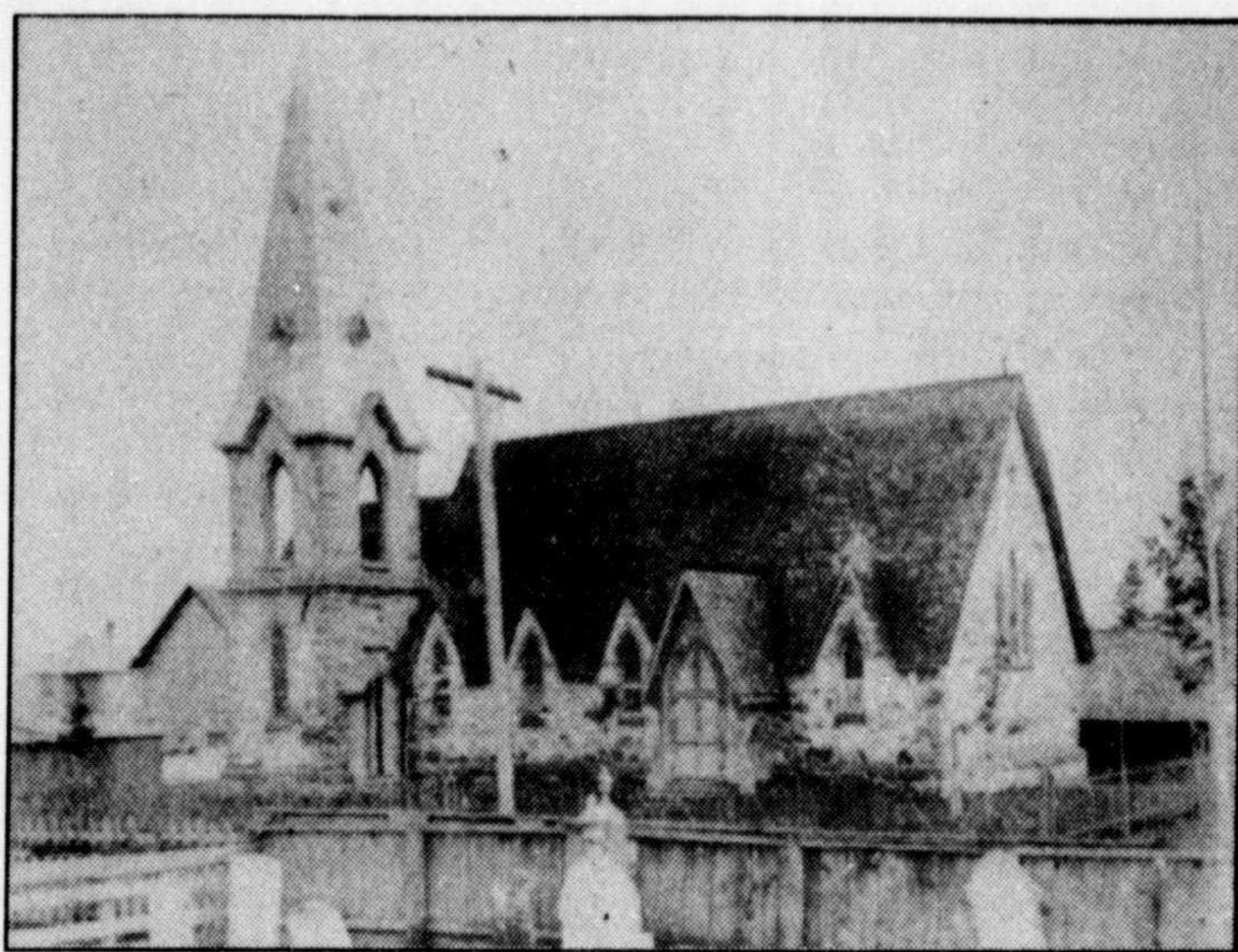
St. Paul's Anglican Church, of which the foundation was laid in 1873. The tower was later reconstructed to support the weight of the bell.
