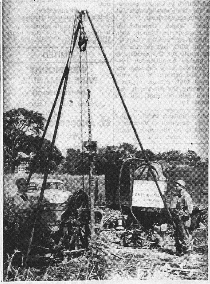
A CREW of foundation investigators are at work on the Nuns' Farm lot between Western avenue and St. Catherine street W. In this case they are drilling to an approximate depth of 40 feet in order to classify the condition of the sub soil in regard to density, water content and compressibility. This information is important in determining the type of structure best suited for the land. (Harrison Photo)
