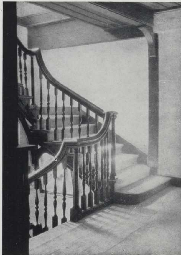
First-floor Landing of the Stair
