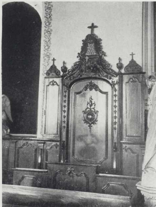
St. Roch. Sanctuary Panelling
