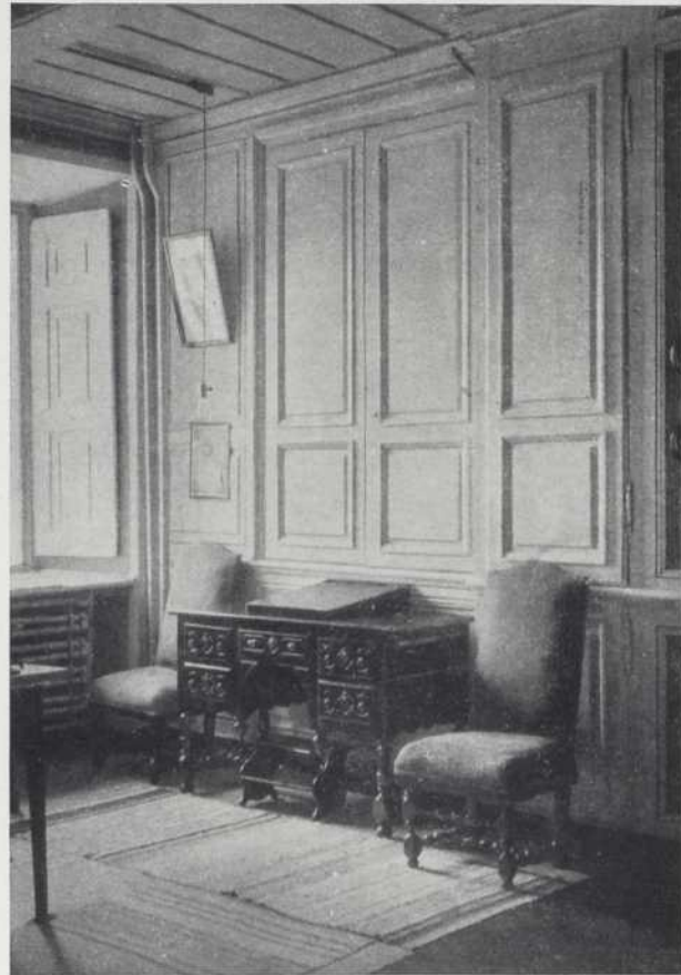
Panelling and Presses
