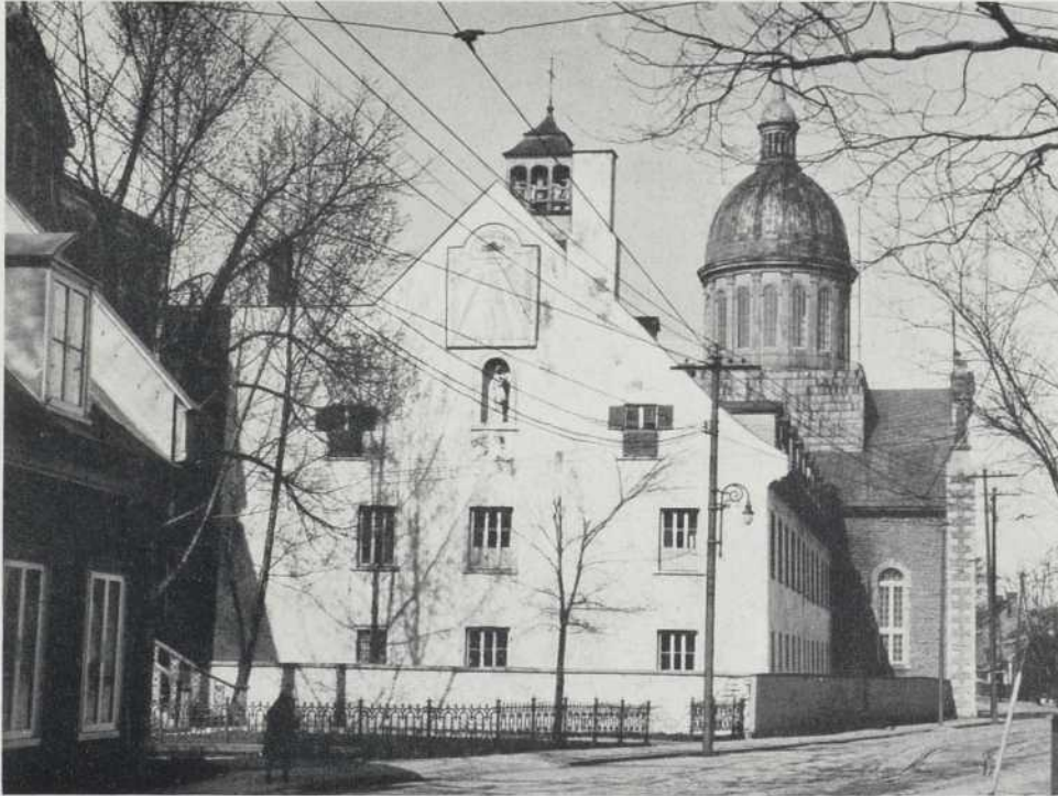
The West Gable
