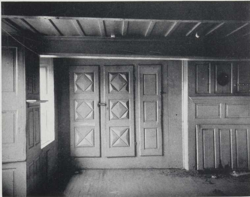
Room in House at Pointe St. Jacques, near Senneville
