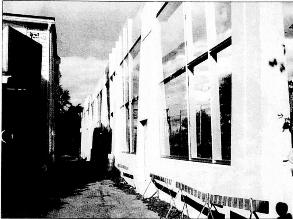
Just a few more panels are needed to finish the experimental barrier.
