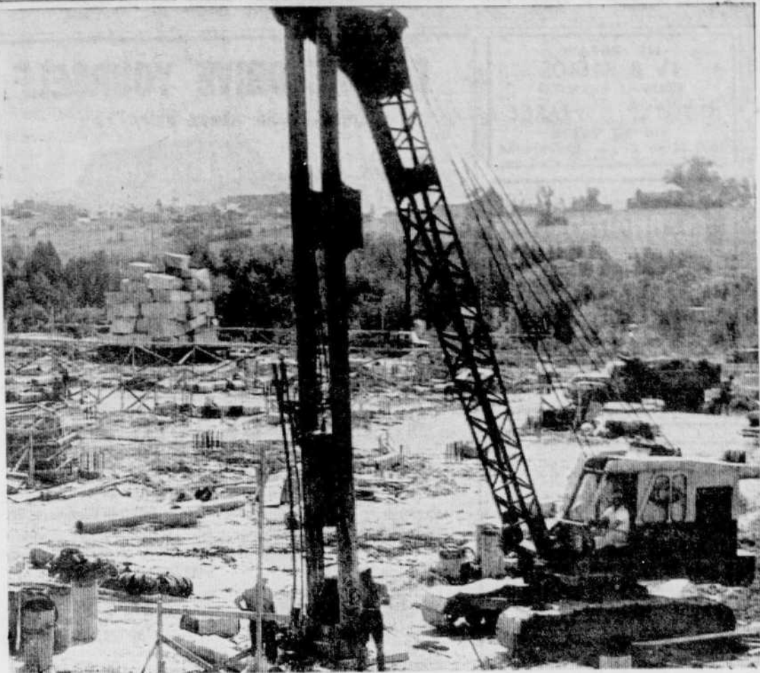
LOWERING THE BOOM — The 35-foot boom pictured above with a drop hammer is driving piles to form the foundation of the new Lowney plant. Some sectional piles are shown to the left front of the picture. A test pile is shown in the background.
