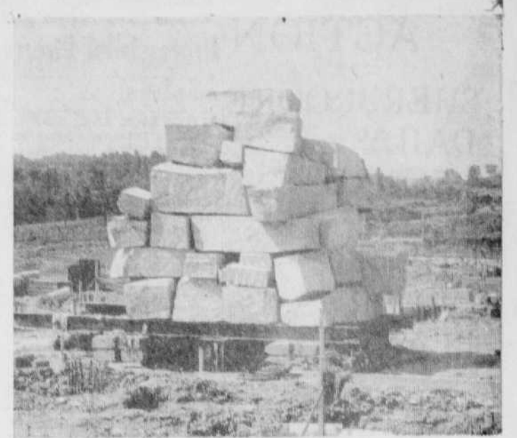
PILE TEST — Shown above are 223 tons of granite, reaching 28 feet into the sky on a platform of steel beams. This load is used to measure the weight the pile will stand without moving. Net settlement of this particular pile was two-tenths of an inch.
