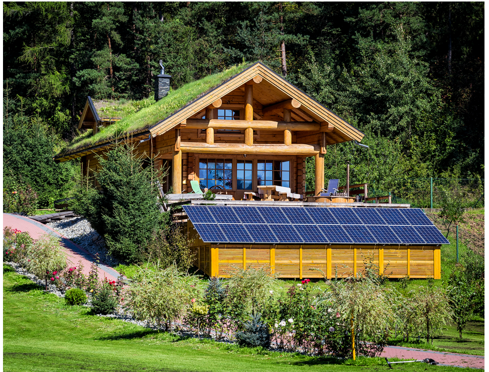
Figure 36. Home located in a remote location and powered by a stand-alone PV system for ac loads.
