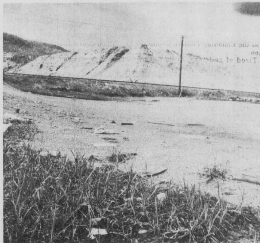
Untouched Eustis tailings dump (top) presents a moderate danger to the environment and needs work. A similar site at Ascot Corner is safer because it has been covered with topsoil, allowing vegetation to return.
