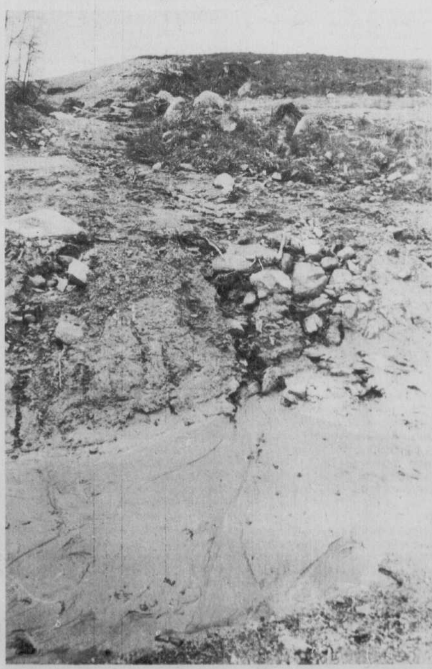
Untouched Eustis tailings dump (top) presents a moderate danger to the environment and needs work. A similar site at Ascot Corner is safer because it has been covered with topsoil, allowing vegetation to return.
