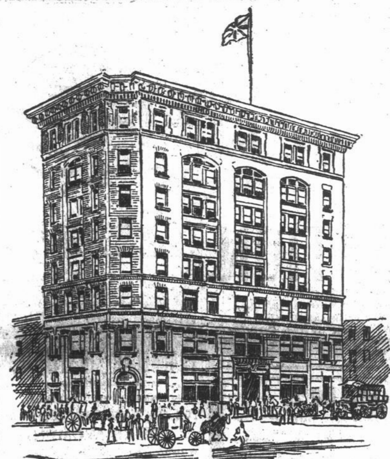
C. P. R. COMPANY'S TELEGRAPH OFFICE BUILDING. Corner of St. Francois Xavier and Hospital streets.
