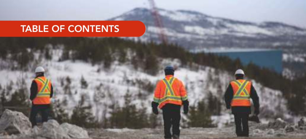
Photo: Nemaska Lithium Inc.
