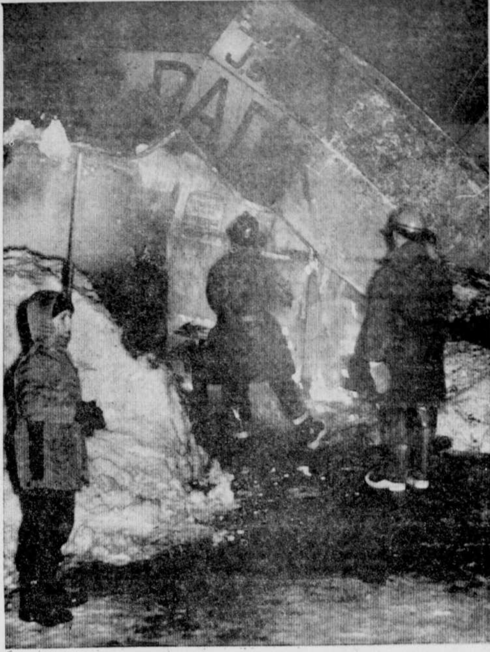
GARAGE FIRE — This is the remains of the Auto Radiator Work garage-workshop at R.R. 1 Rock Forest which was razed by fire late Friday night. The structure, belonging to Robert Cloutier, was completely demolished. Flames spread from a defective wiring system, Mr. Cloutier said. The owner estimated damage at $15,000. (Record photo by Doug Gerrish)
