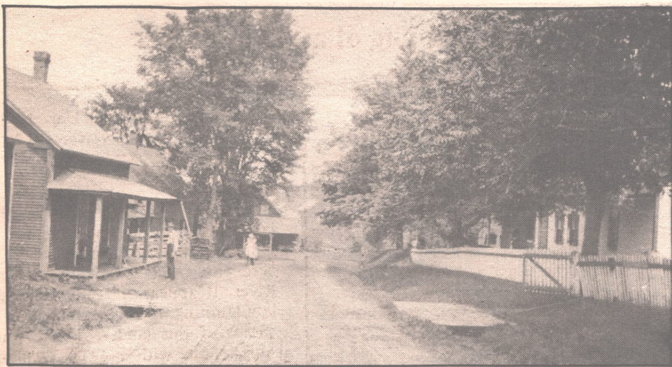
Suitor road looking north towards Grist Mill
