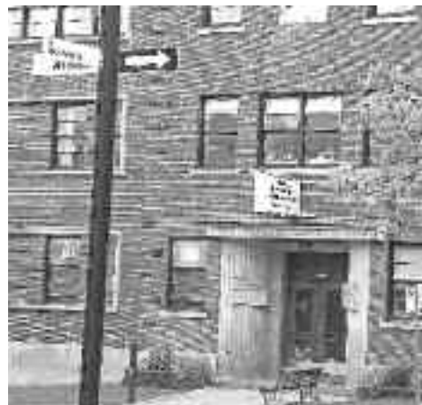
A June 2012 photo of the Gilman Pavilion on Atwater south of Dorchester. Photo: Independent files
