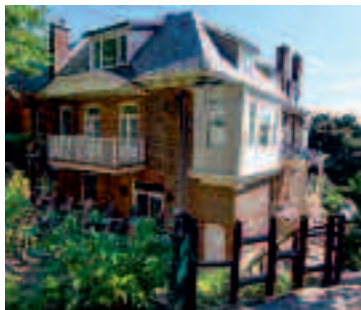
WSMT | THE BOULEVARD LOVINGLY RESTORED
