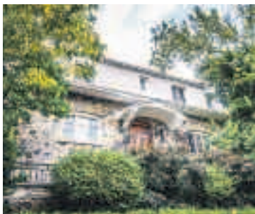
WSMT | EDGEHILL ROAD CONTEMPORARY DETACHED
