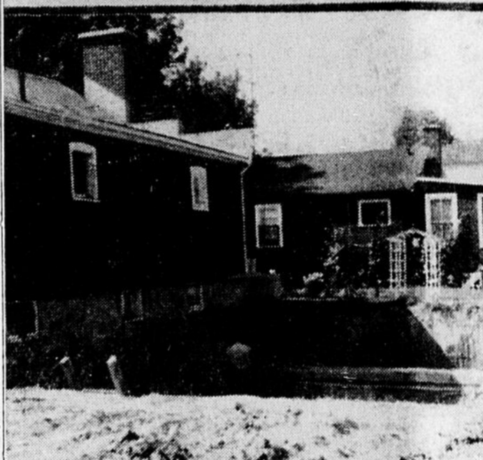
Top photograph shows the Canadian Legion Hall at Ormstown with front entrance to same. This hall is well used throughout the year and of late has been rather crowded for space. Thus an addition is being made and the lower photograph shows the excavation at the side where this new addition will be made. The article below explains more fully what is proposed will take place.
