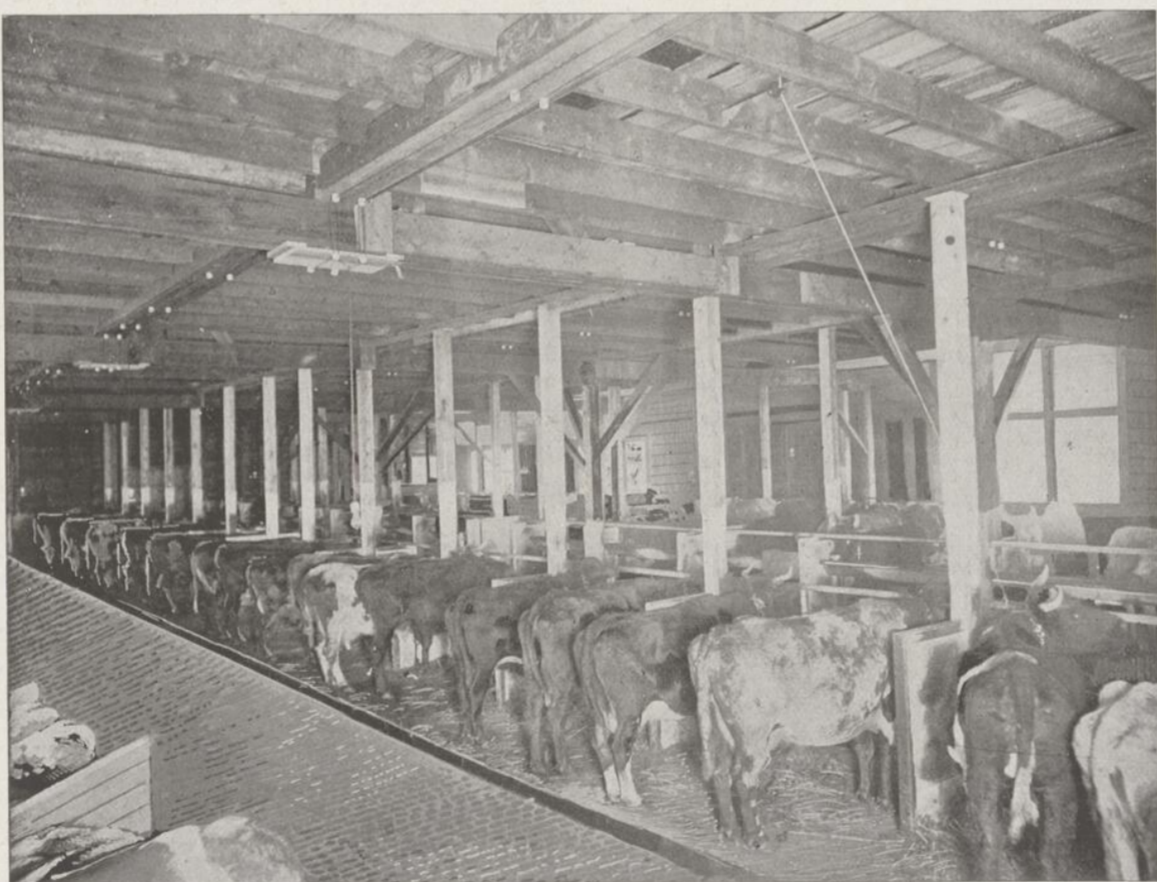
INTERIOR OF COW STABLE.
