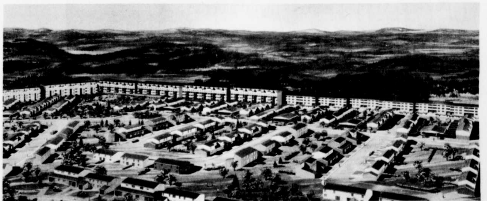
NEW TOWN DESIGN — Fermont, the new community being designed and built for Quebec Cartier Mining
