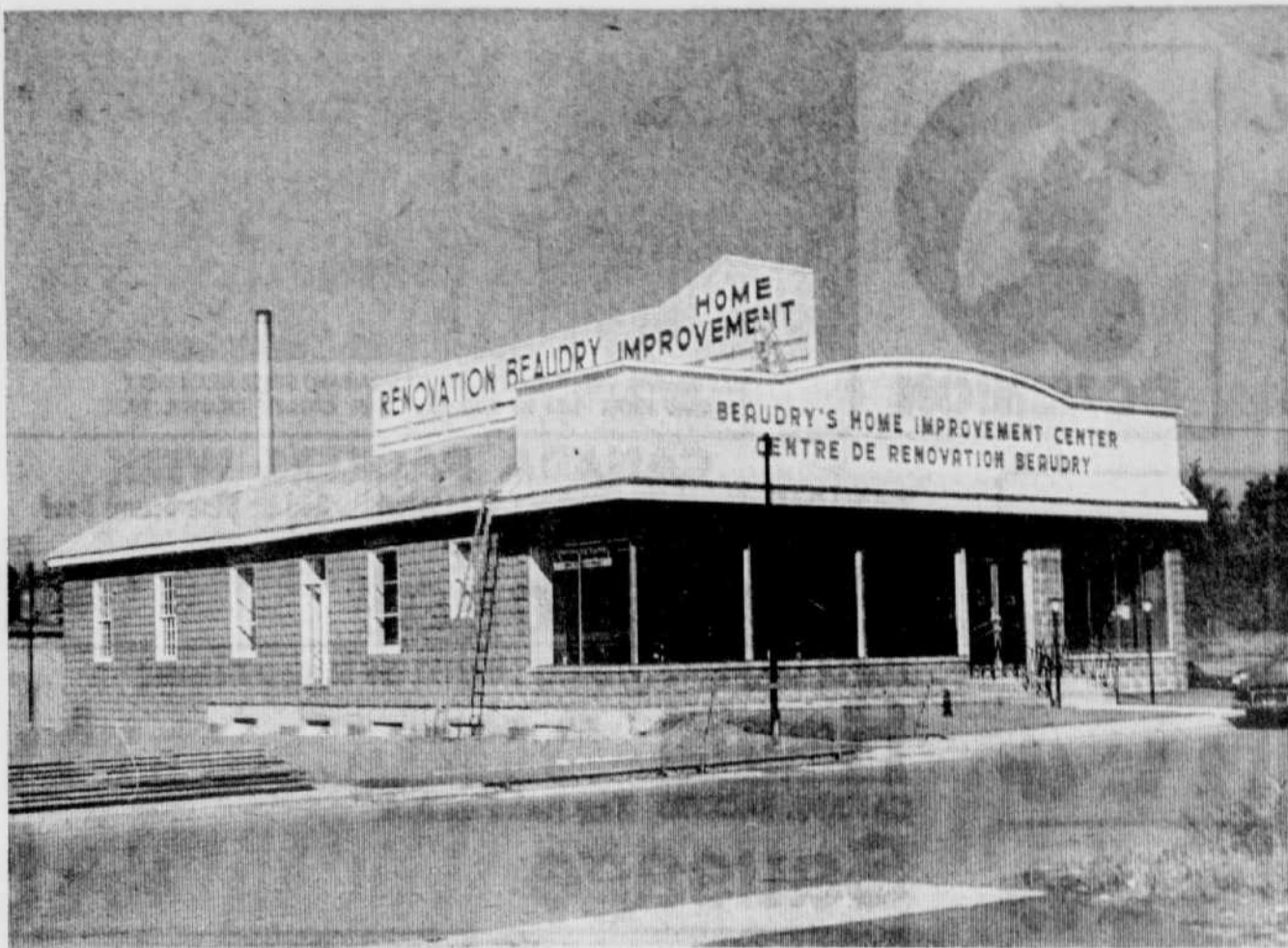
Beaudry's Home Improvement Center (Division of Beaudry Lumber Inc.) situated at the corner of King West & Bryant, Sherbrooke
