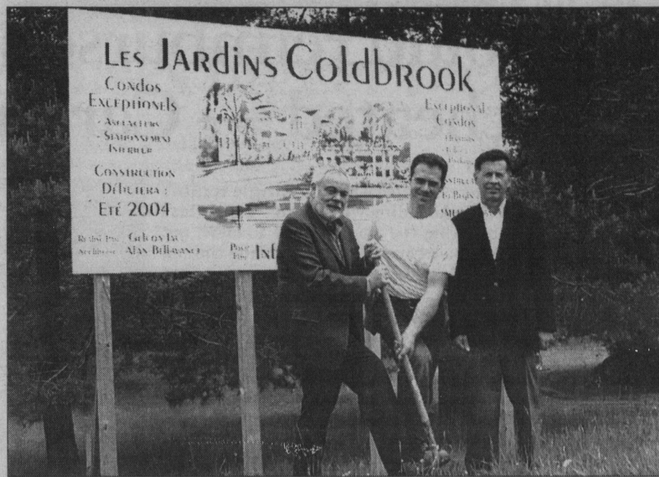
Brome Lake mayor Richard Wisdom joined Philippe and Gaëtan Gélinas for the ceremonial first shovel of earth at Les Jardins Coldbrook Monday. Over the next three years a total of 72 condos will be built in the development, an investment in excess of $10 million.
