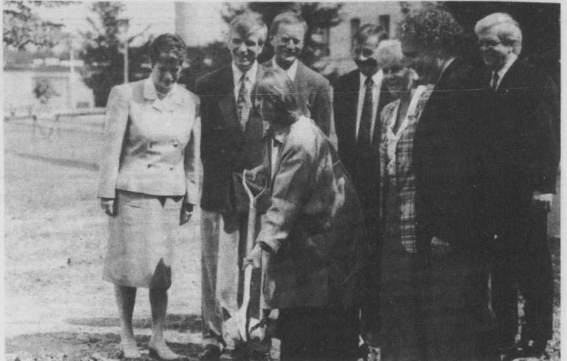
Dignitaries turn the soil for the new clinical research facility
