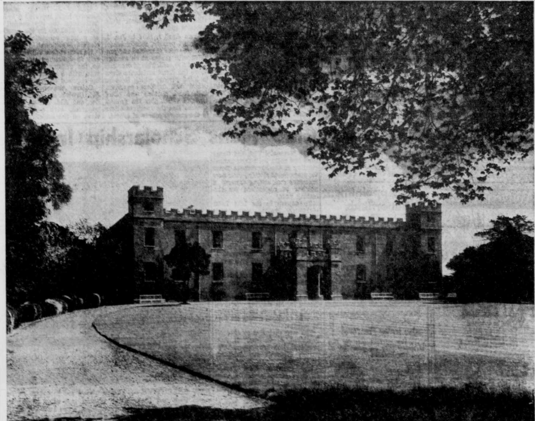
ONE OF THE STately HOMES OF ENGLAND, SYON HOUSE, BRENTFORD, HOME OF THE DUKE OF NORTHUMBERLAND
