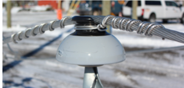
Tie wires in good condition
