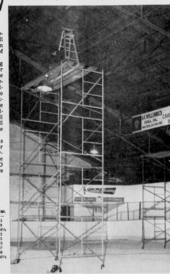
IS RENOVATED — Workmen are seen as they work on the Waterloo Arena installing a new system of lights. The sum of $5,020 is being spent in renovating the inside of the Arena. It is hoped the job will be completed for Saturday in order that ice may be installed. (Record photo: Marcel Cote)
