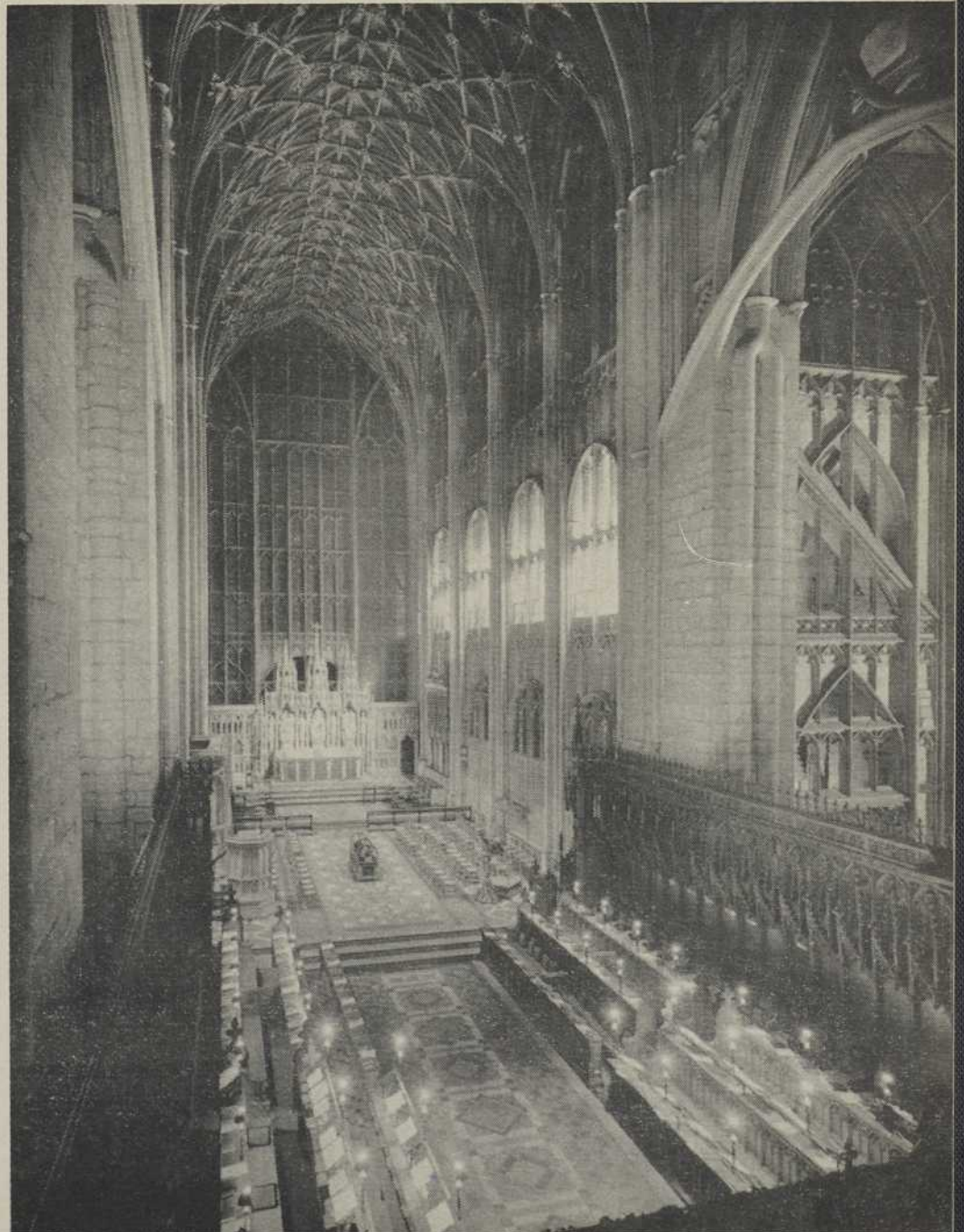
CHOIR ILLUMINATED SHOWS THE DECORATIVE WROUGHT IRON DESK LIGHTS.
