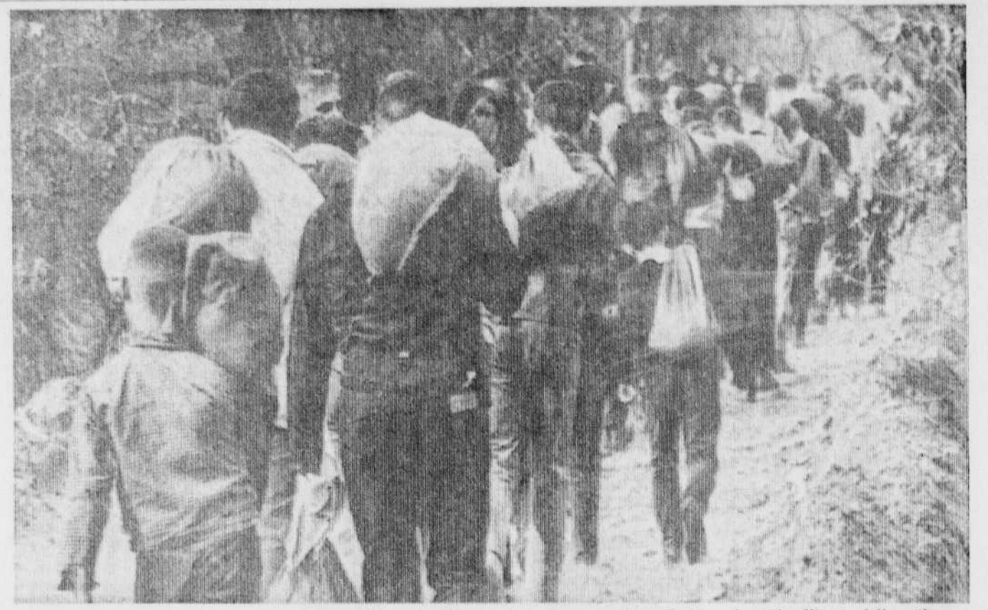
UNDETERRED — When seepage under a dike cut off access to truck delivery, young volunteers shouldered the bags for a quarter-mile hike along the dike to deliver them to a trouble spot at La Crosse yesterday. (AP Wirephoto)
