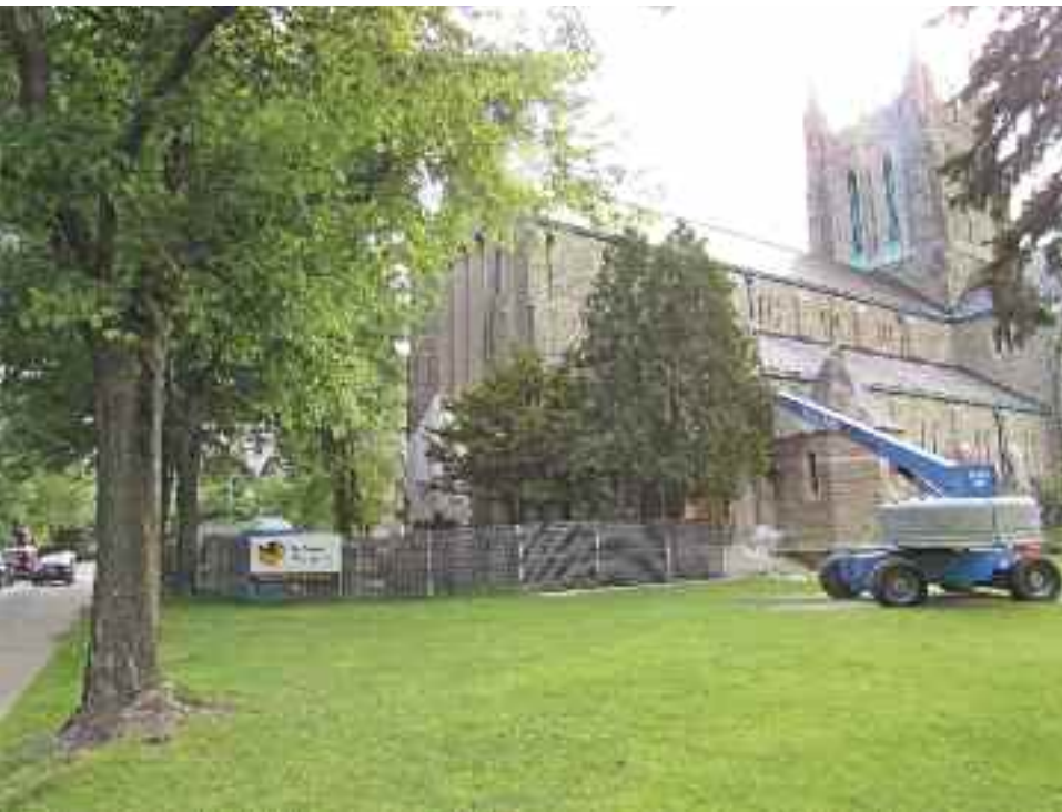
The front steps and surrounding masonry of the Ascension of our Lord Catholic church at Sherbrooke and Kitchener received a sprucing-up last week. The work, seen here on June 9, had been completed by June 13, according to Monsignor Sean Harty. Approximately $120,000 will be spent on the project.
