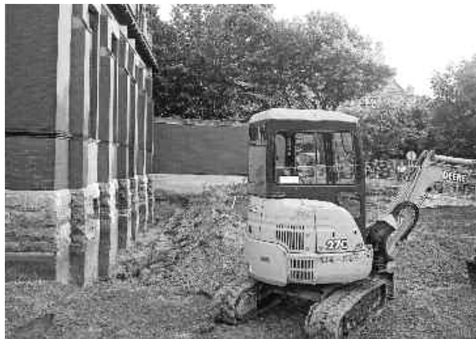
Work began last week to waterproof foundations of the library, seen here along the Sherbrooke St. façade looking west.
