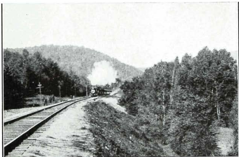
THROUGH THE EASTERN TOWNSHIP HILLS, NEAR SHERBROOKE, QUE.
