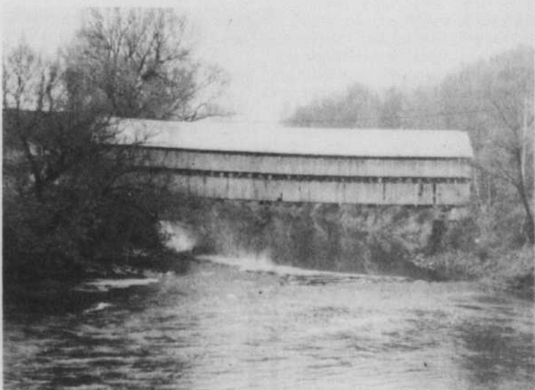
This one, built in 1870, crosses the Massawippi River at Capelton.
