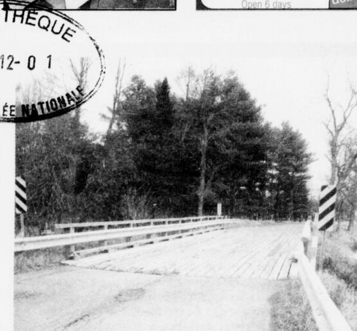
The Cowan bridge in Havelock, which spans the English River, will have a whole new look in four months. (photo PL)
