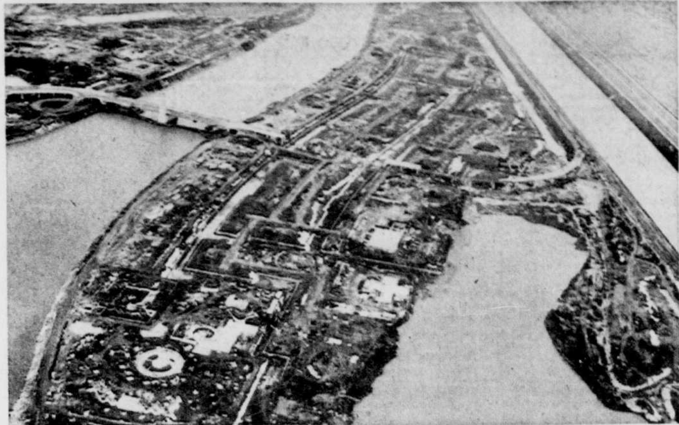
WORK PROGRESSING — Aerial view of Ile Notre Dame and Ile Ste. Helene shows construction work under way on nearly all Expo 67 pavilions. The circular foundation is that of the Canadian pavilion, the cross-shaped one that of Quebec, and immediately behind that the French pavilion. The most advanced building, the Scandinavian pavilion, is on Ile Ste. Helene near the bridge. (CP Photo)
