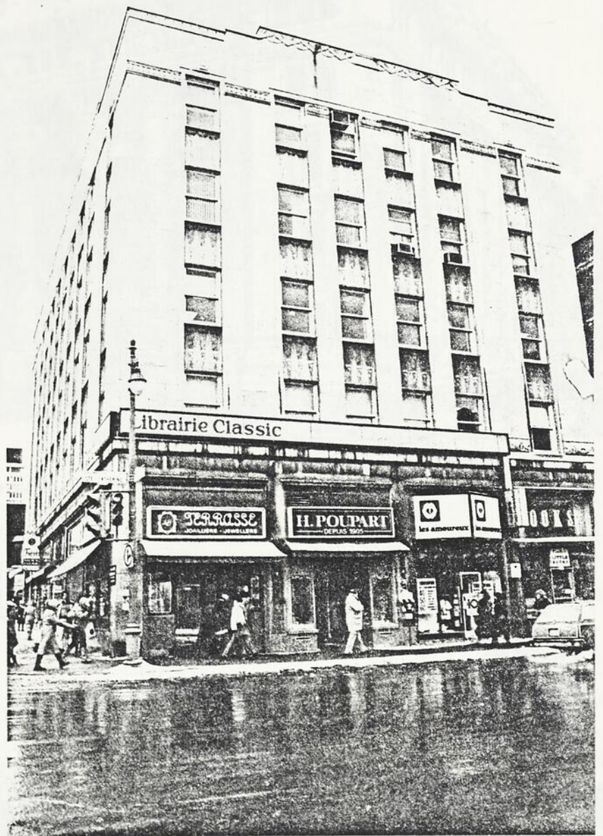
Fig. 248 Edifice Crescent, 1327-33 Sainte-Catherine O.
