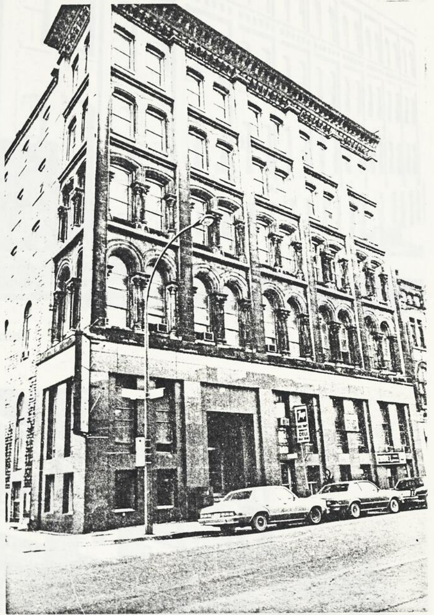
Fig. 258 Mercury Building, 651 Notre-Dame O.
