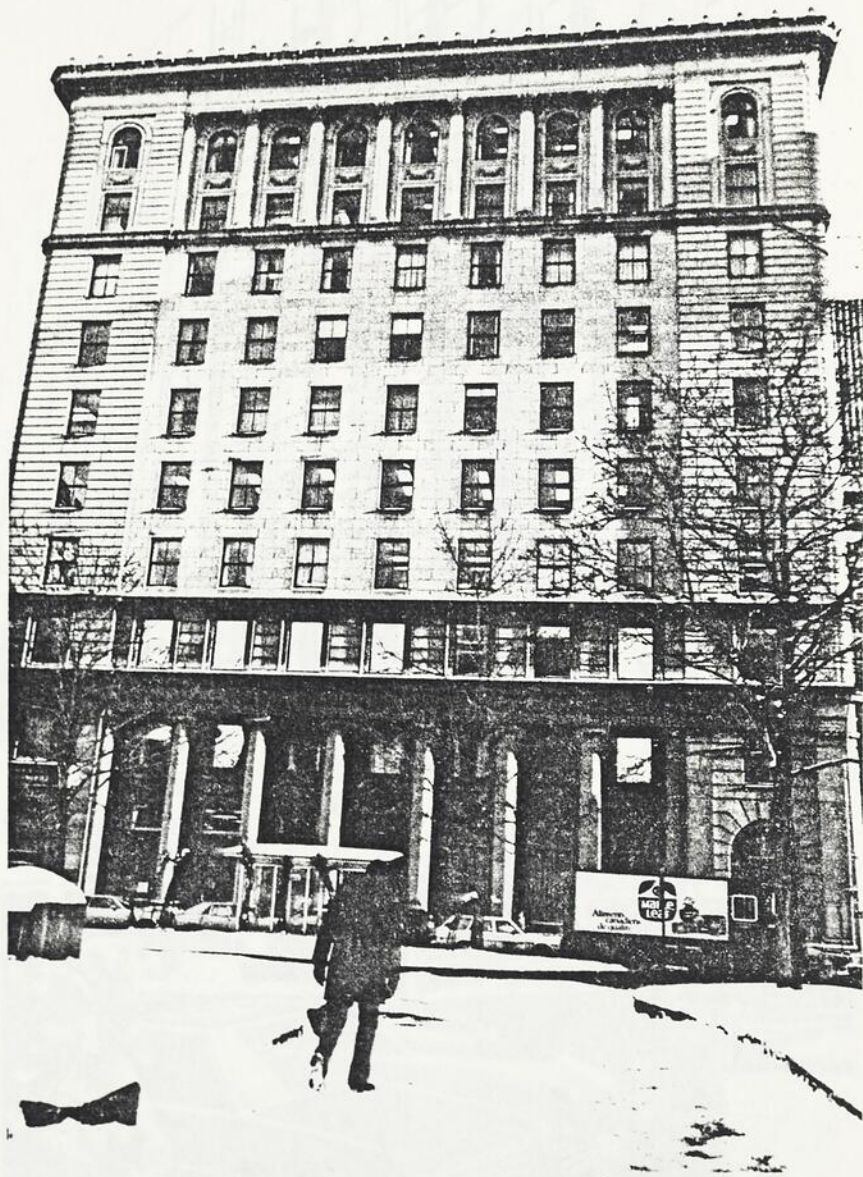
Fig. 246 Canada Cement Co. Building, 606 Cathcart.
