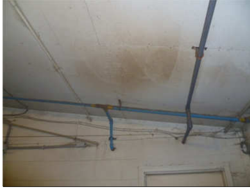
Figure 25 The perimeters of these propane pipes must be sealed with an appropriate caulk (Flextra)
