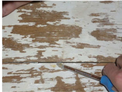
Figure 20 Joint between two plywood sheets that has to be sealed
