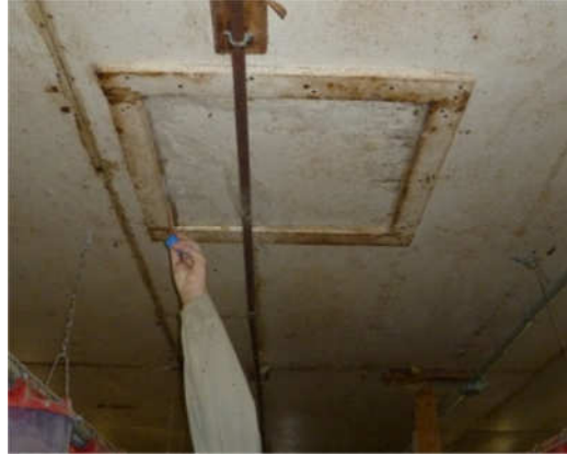
Figure 48 Attic access hatches blocked off
