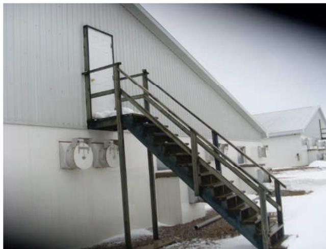
Figure 9 Example of attic access from the outside
