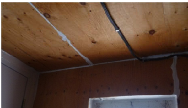
Figure 21 Caulk applied along the joints between plywood sheets
