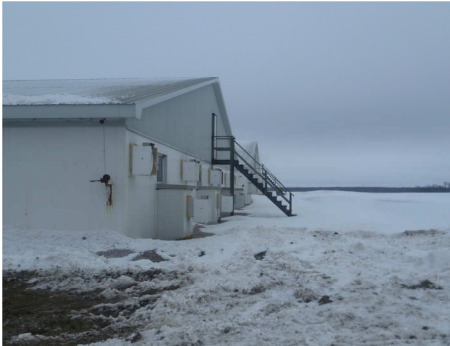
Figure 49 Attic access by the exterior of the building
