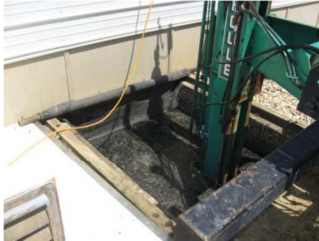
Figure 46 Canvas curtain hanging onto the manure surface to minimize air infiltration Photo: Darwin Reicks
