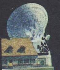
STATION TERRESTRE INTELSAT STANDARD "A" Première Installation 1963
