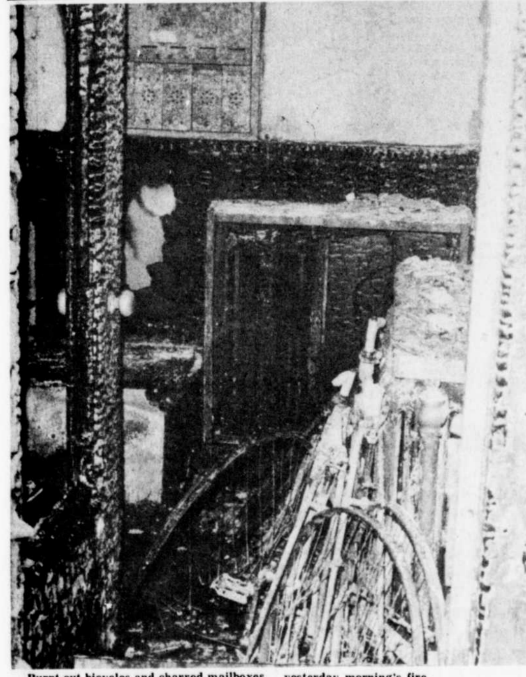
Burnt-out bicycles and charred mailboxes mark the entrance to the Frontenac St. apartment building where two died in yesterday morning's fire. (Record Photo by Bruce Porter)
