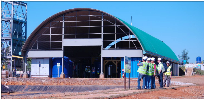
Figure 5.60: Leach solution processing plant.
