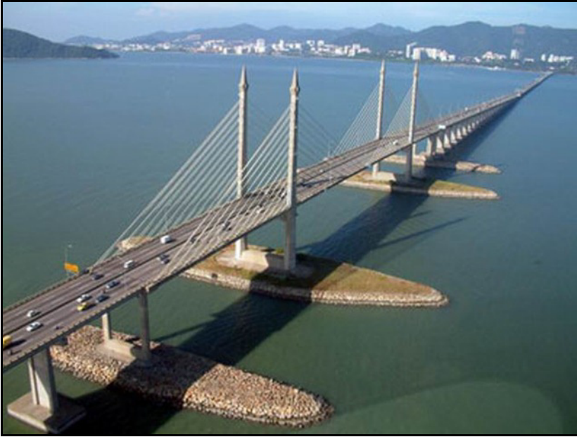
Figure 4.5: Penang Bridge is 13.5 km long opened in 1985.
