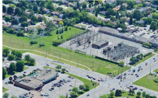
Photo 1 – Aerial View of Existing Saint-Jean Substation
