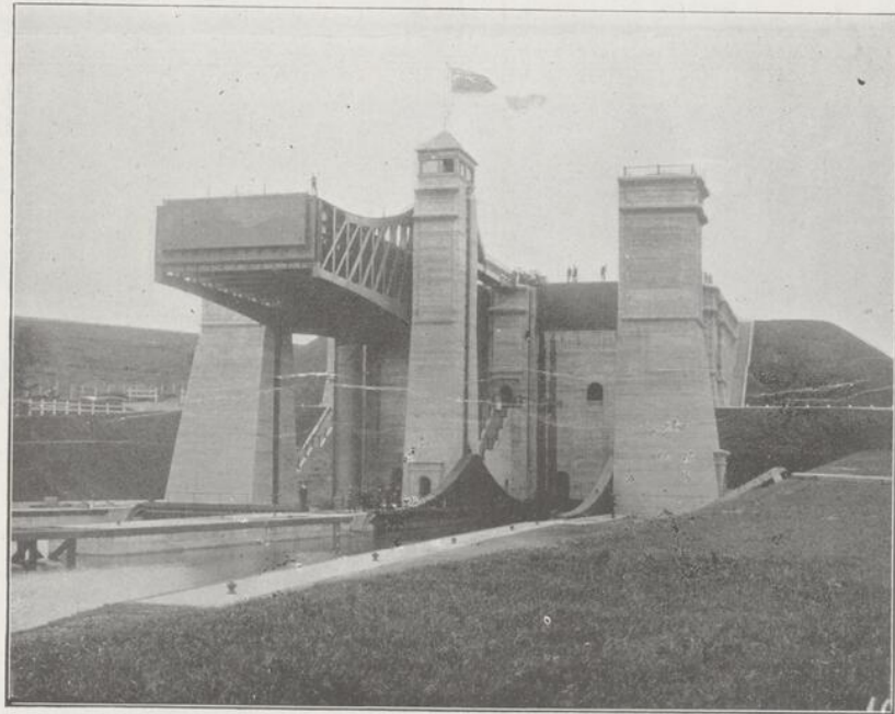
LIFT-LOCK AT PETERBORO—This is the largest lock of its kind in the world, and forms a link in the Trent Valley Canal project. Some time ago serious defects, demanding a Government inspection, were discovered in its construction.
