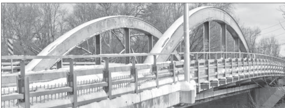
The Bishop's Bridge in 2013 (Courtesy of Mark McLaughlin)
