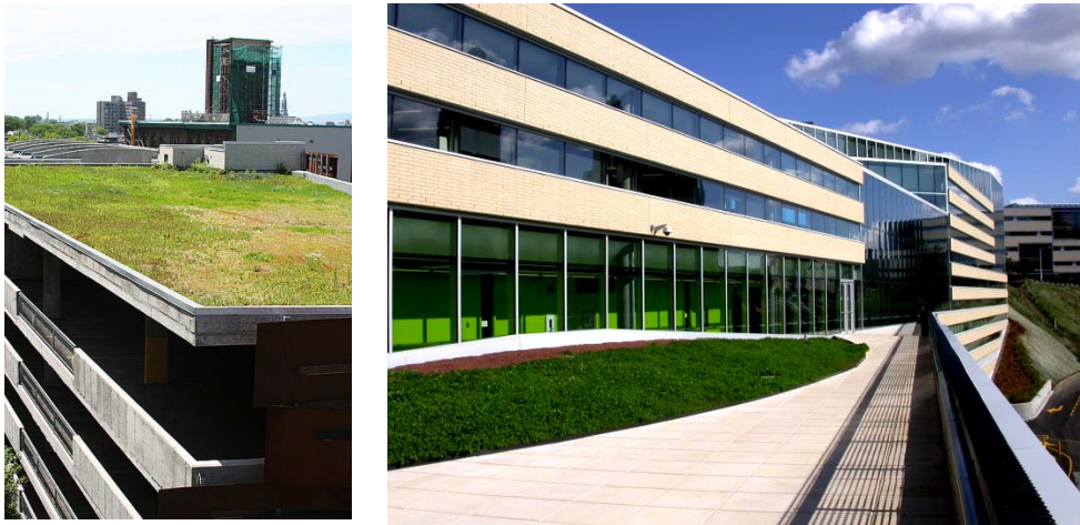
Figure 5 Extensive green roofs
