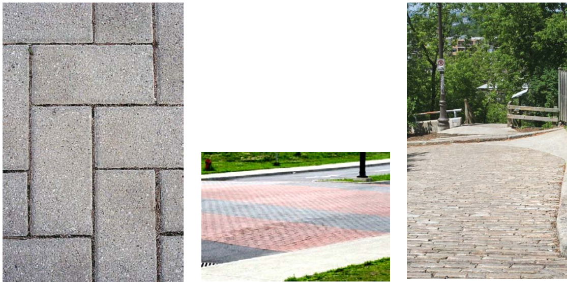
Figure 7 Impermeable paving stones with permeable joints. Pedestrian areas with paving stones that allow water percolation
